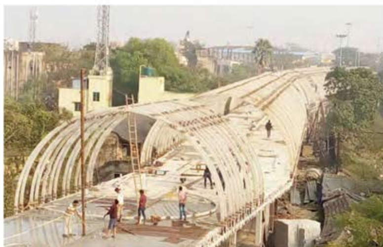
Dakshineswar Sky Walk under construction. Photo: © Design Forum International
