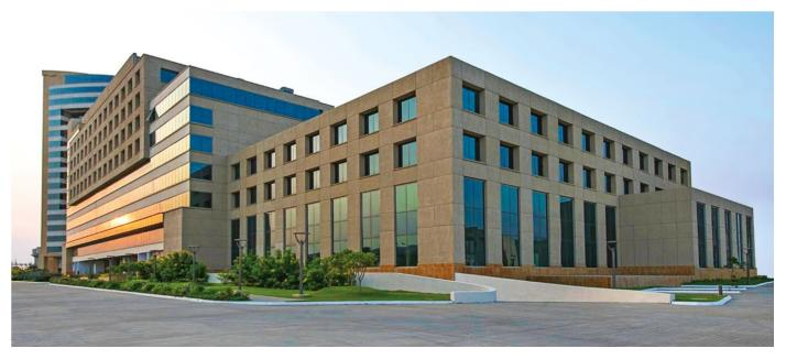
Cyberwalk has a dedicated area of 25,000 sq-ft to 38,000 sq-ft for commercial office space. Since the building aimed at a LEED rating, the architect selected SGG Envision glass, a high performance material with excellent thermal insulation properties and high spectral selectivity. In addition to delivering a superior performance, Envision also enables abundant light transmission and is relatively more transparent than other solar control glasses.
